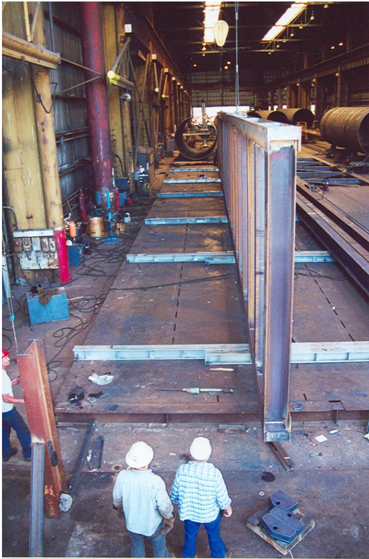
Figure 4 TBS Pipe Pile Fabrication
