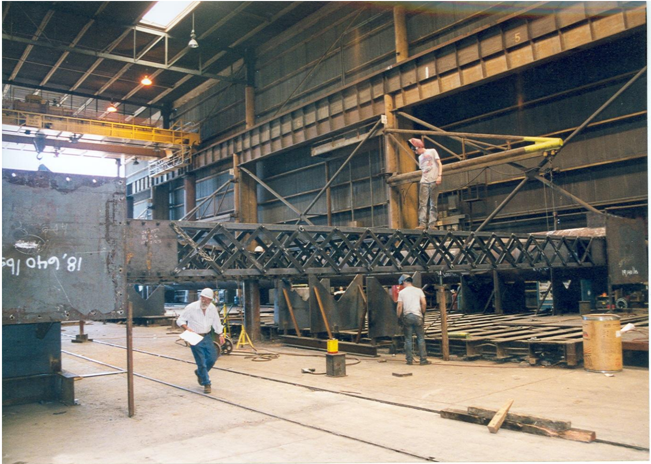
Figure 1 TBS Fabrication Shop
