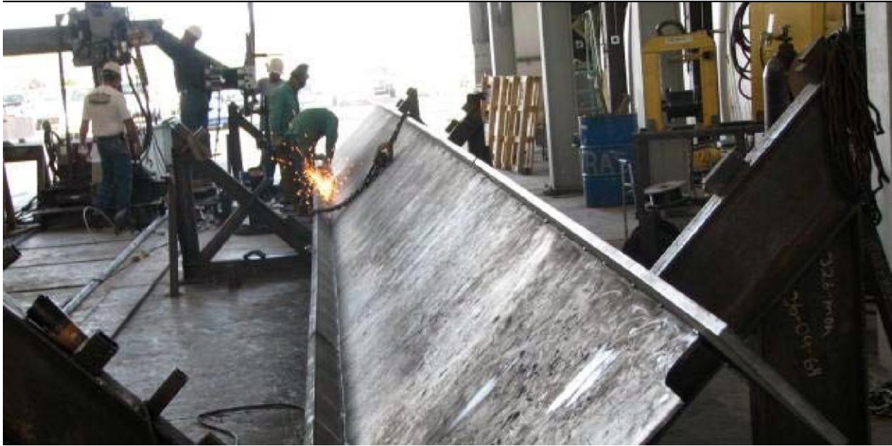
Figure 9 Girder Fabrication at Stinger Welding
