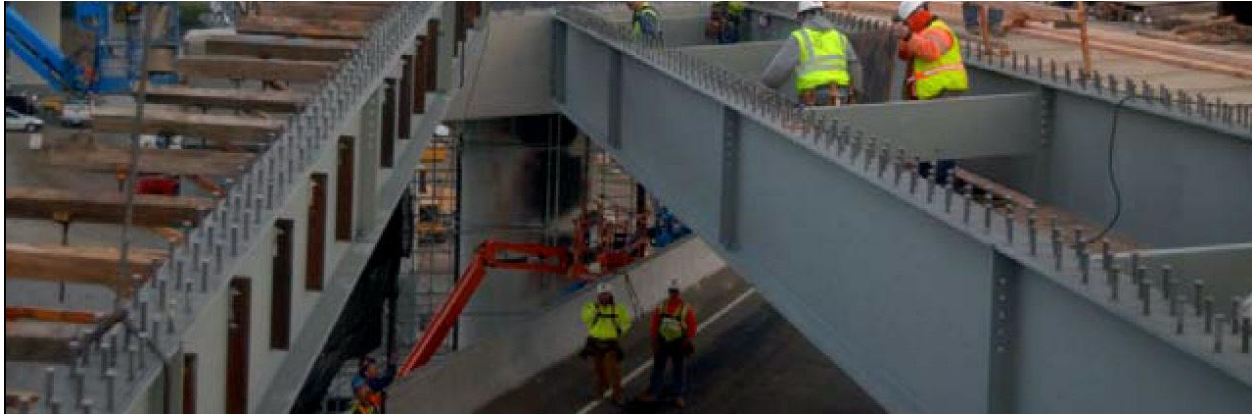
Figure 10 Erecting Final Replacement Girder at MacArthur Maze
