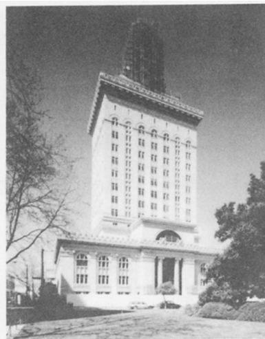
Figure 1: Oakland City Hall
