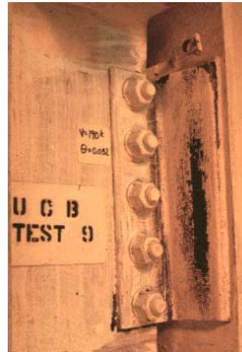
Figure 2.3. Failure of Weld
